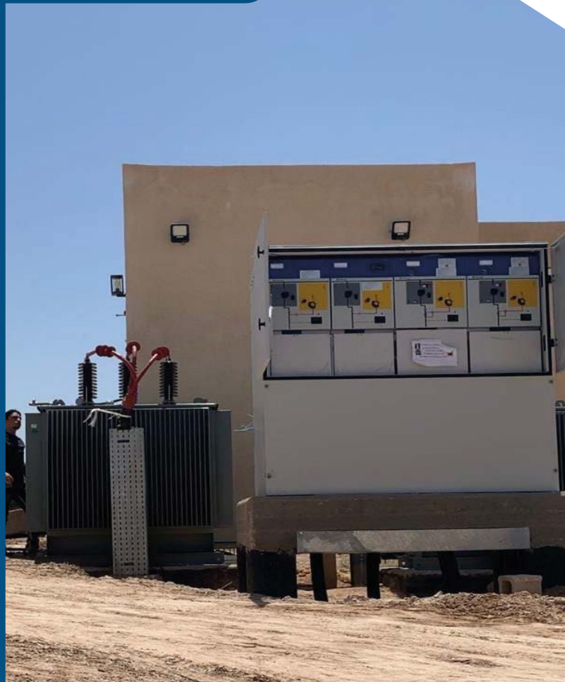
Balqa University Project
